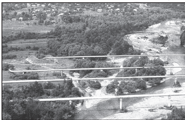
Fig. 7.17: Pipelines transporting natural gas in Ukraine
