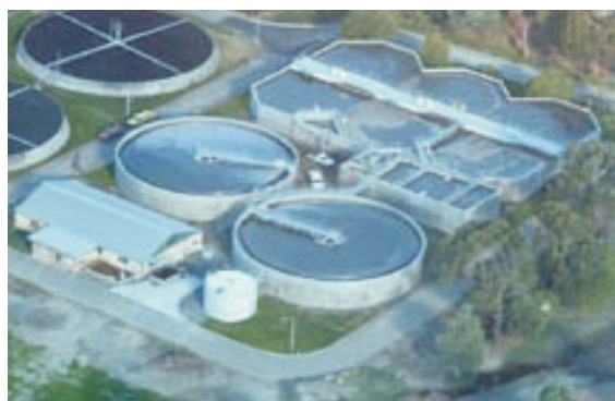
Figure 8.7 An aerial view of a sewage plant
